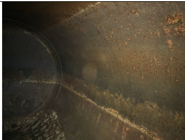
Pitting along upper wall and roof
