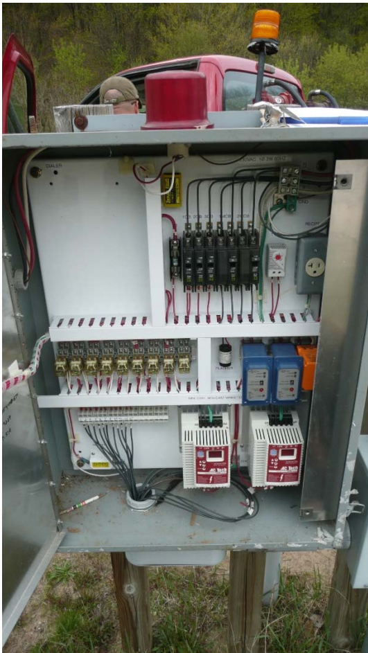
Control Panel interior
