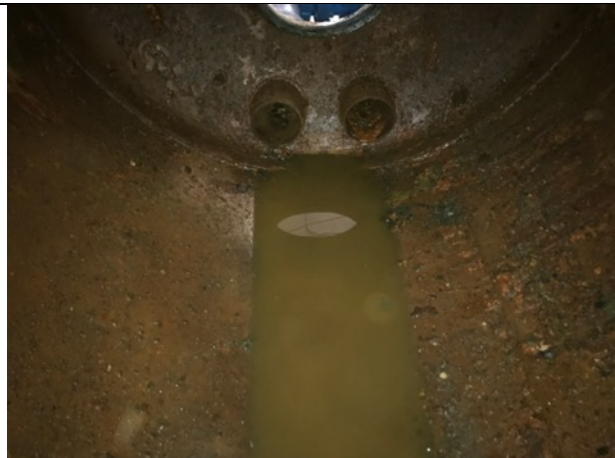
Inlet and outlet piping on east head
