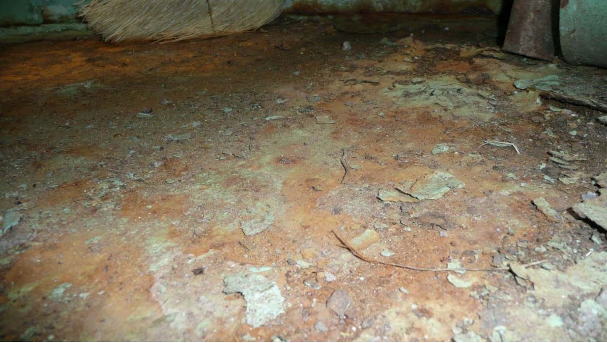
Poor condition of can floor
