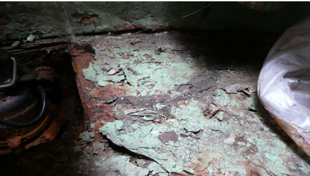
Can floor steel delaminating near sump
