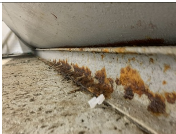
Corrosion on steel chock block
