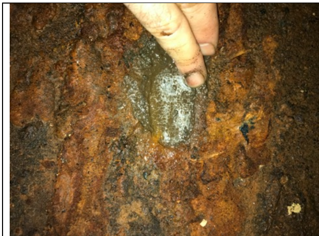
Deep pit on wall
