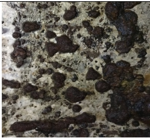
Pitting on walls
