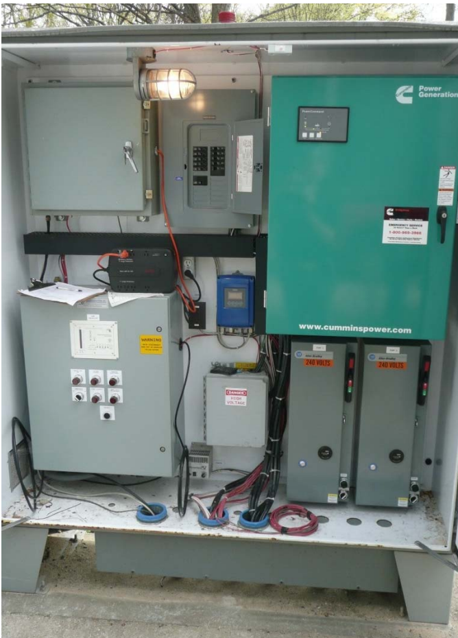
Electrical and Control Panel interior
