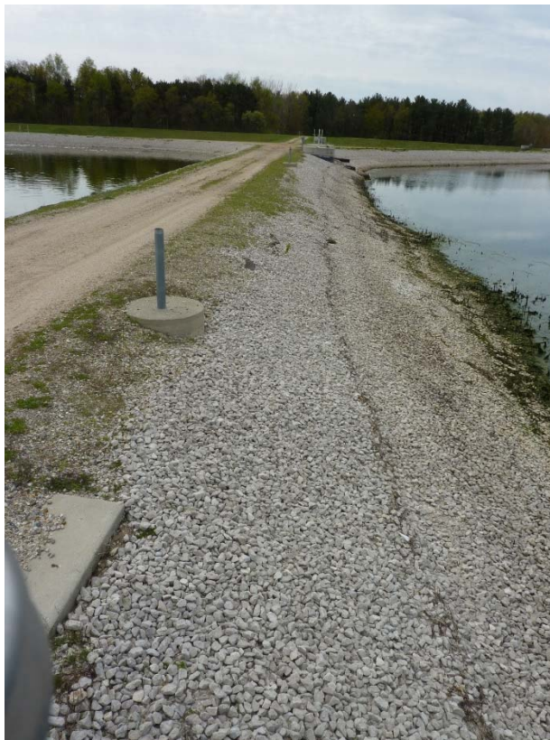
Lagoon No. 2B berm in good condition (facing south)
