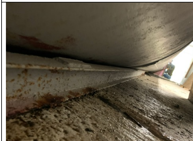
Corrosion on steel chock block
