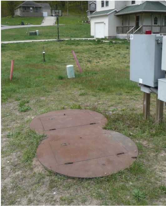
Lift Station Site
