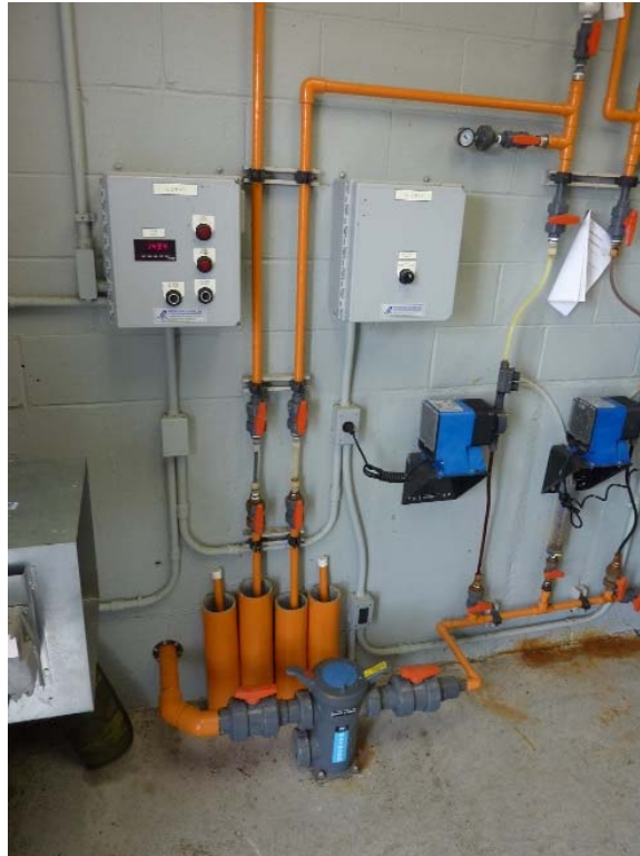
Level sensor display, basket strainer, metering pumps
