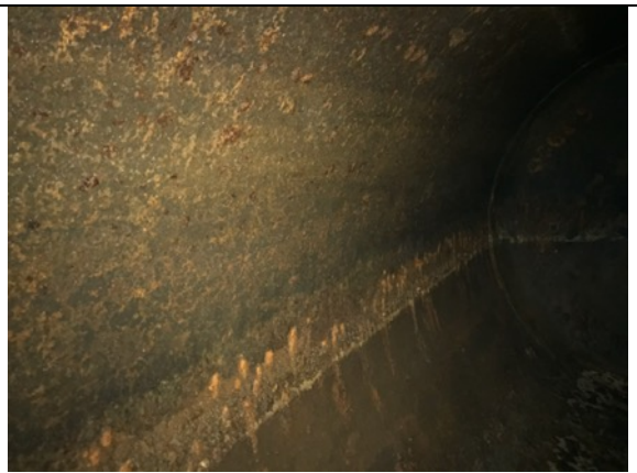
Pitting along upper wall and roof
