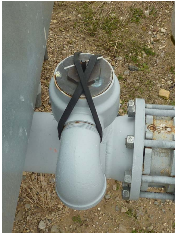
Lagoon No. 1A air header and berm (good condition) Blower No. 2 failed air relief valve
