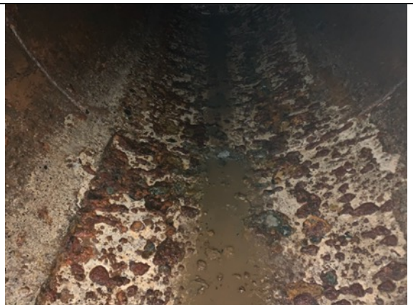
Heavy pitting on floor
