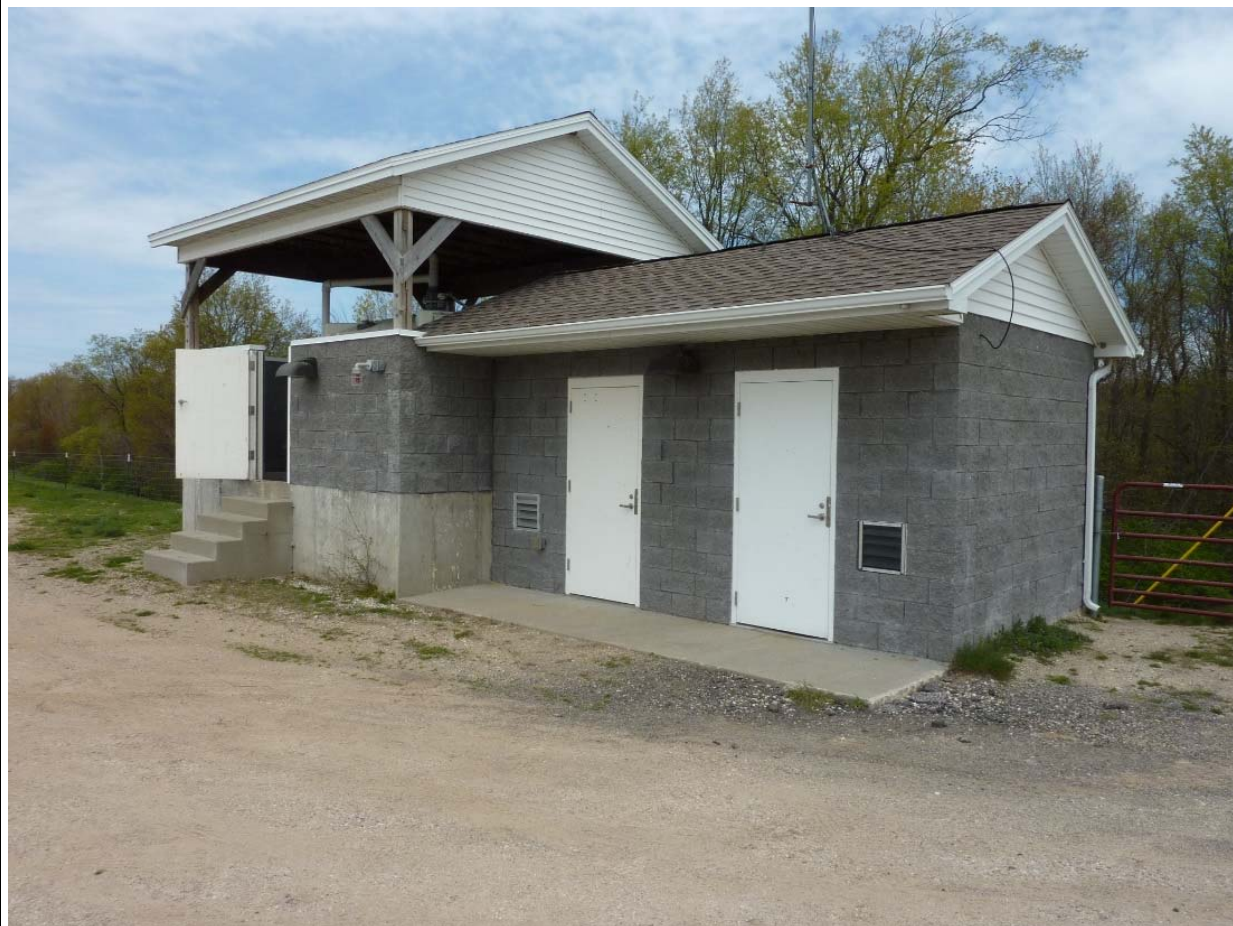
Ferric chloride storage system and Treatment Building
