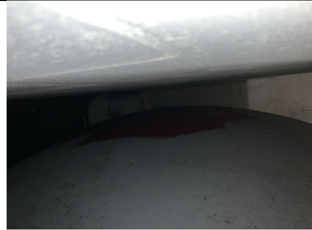
Western head with only primer coat at center
