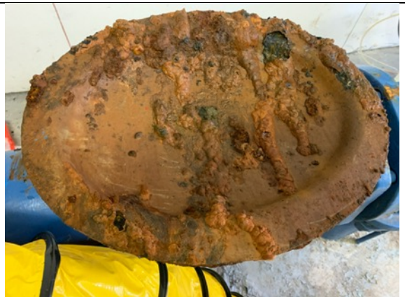
Deep pitting on interior side of manway hatch
