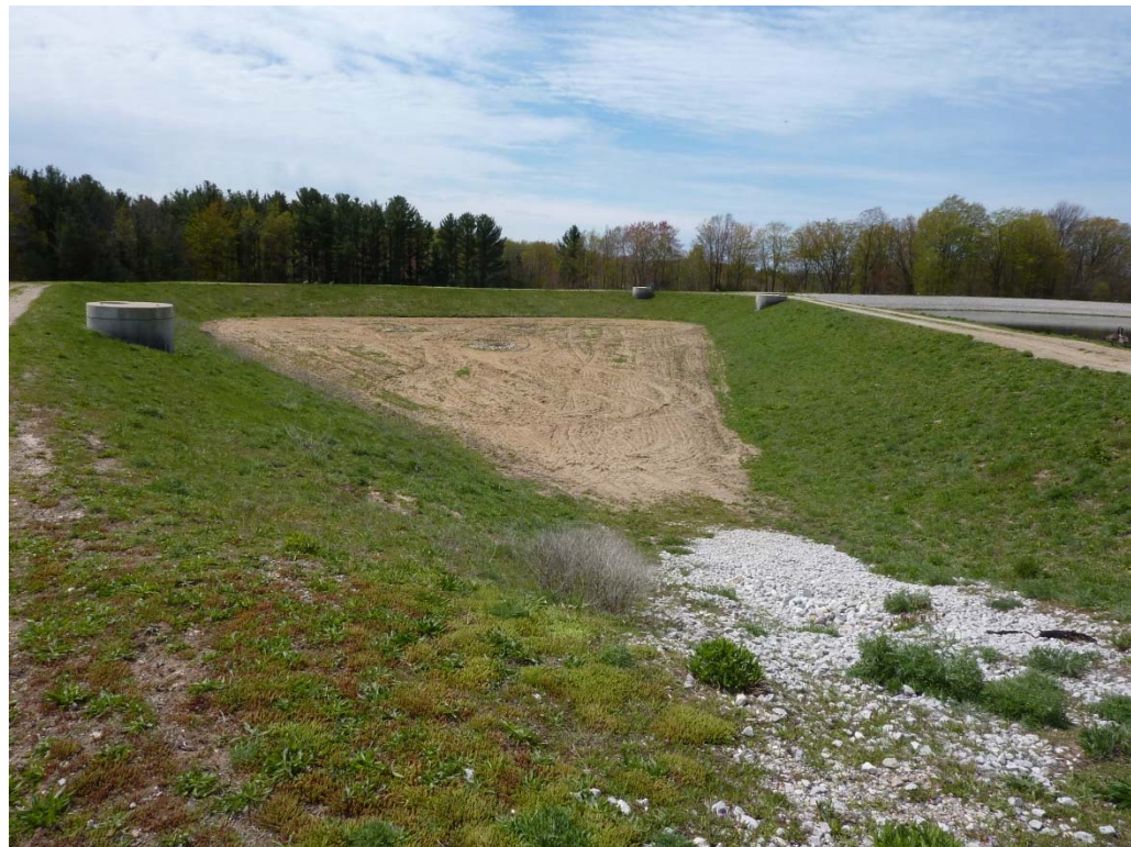
RIB No. 3 (facing southwest)
