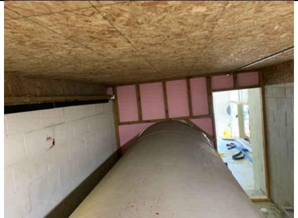
Top of tank with chipping of top coat
