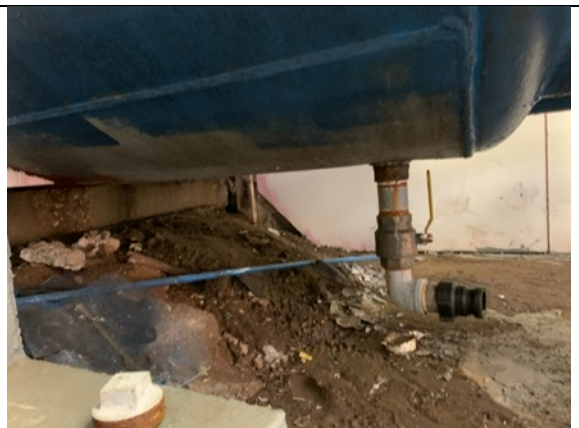
Drain at bottom of tank
