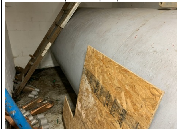
Topcoat is chipped in a few locations
