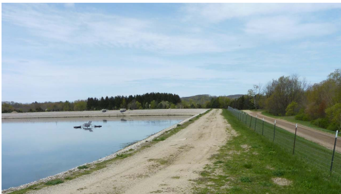
Lagoon No. 2A and Lagoon Circulator (facing west)
