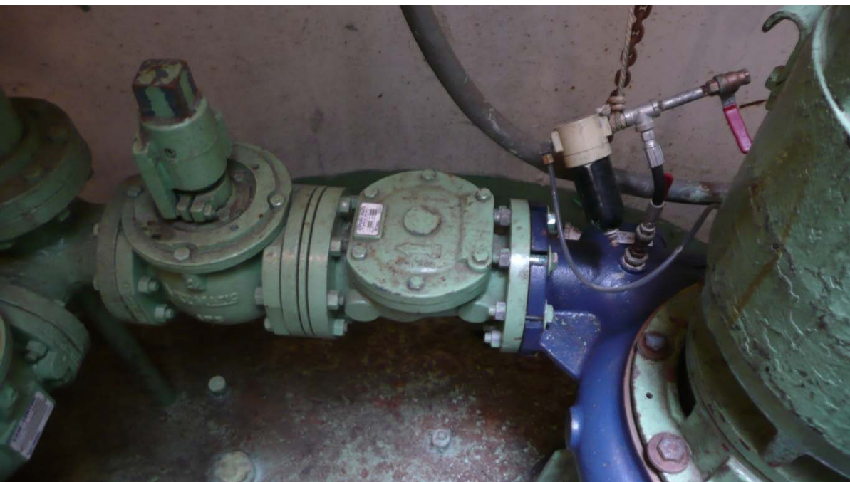
Discharge Check and Isolation Valves
