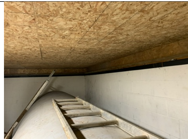
Top of tank in annex room
