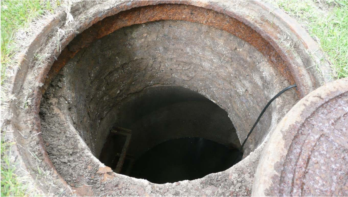
Wet Well with misaligned manhole and riser missing mortar between bricks
