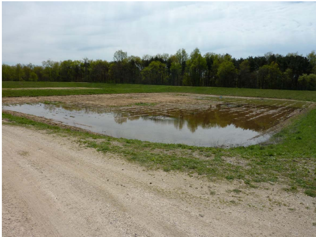
RIB No. 2 in use during condition assessment (facing southeast)
