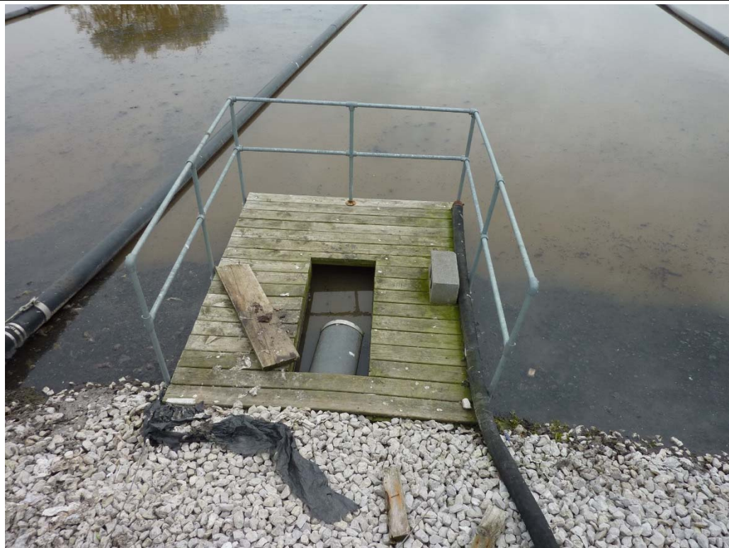
Lagoon No. 1A2 overflow pipe to MH#1
