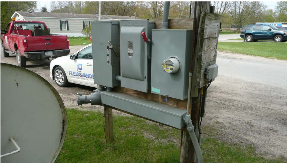
Electrical equipment and meter
