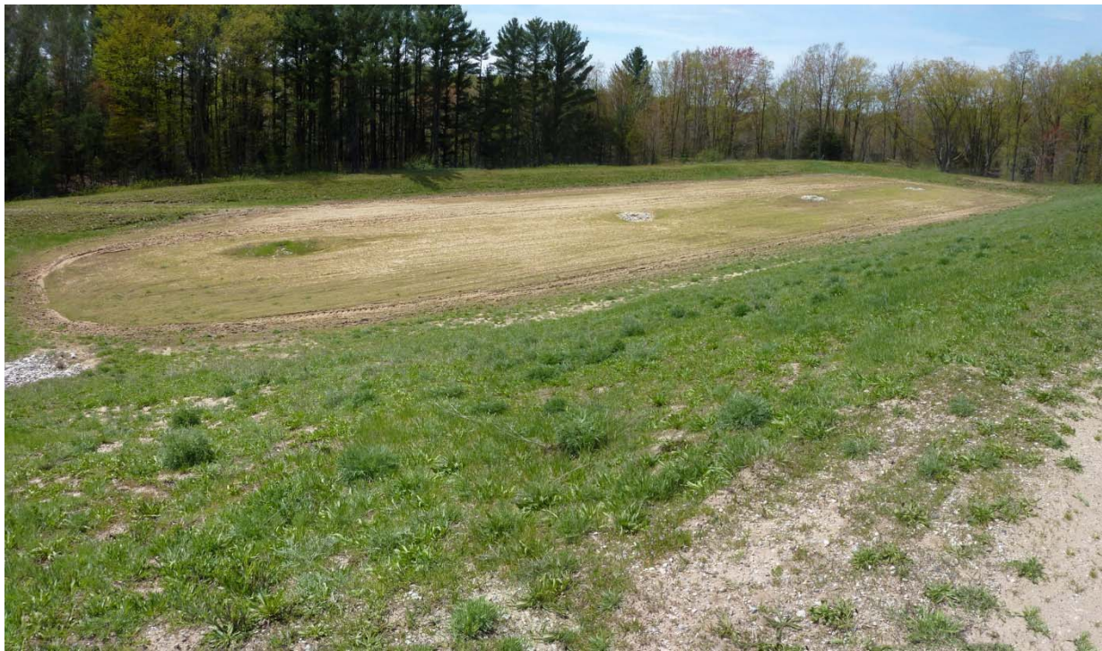
RIB No. 3 (facing southwest)
