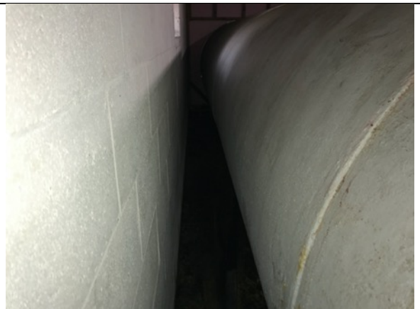
Back side of tank
