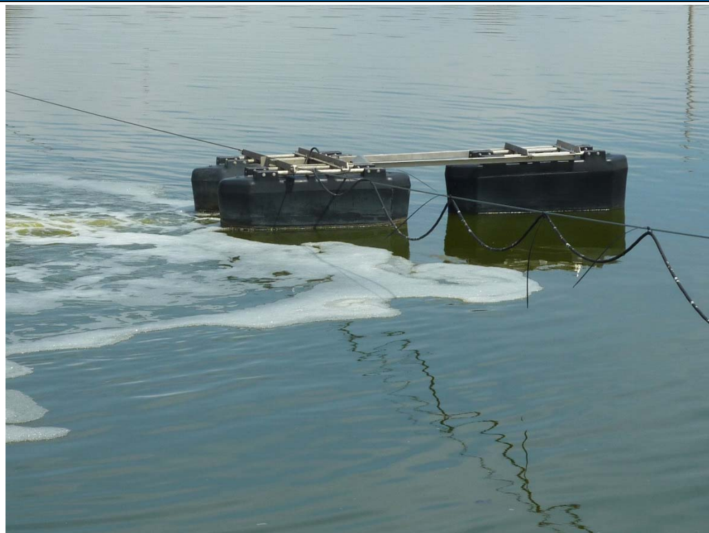
Aspirating Aerator No. 1 in Lagoon No. 1B
