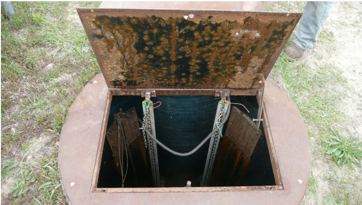
Wet Well hatch in poor condition (typical of both hatches)
