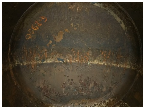
Pitting on western head
