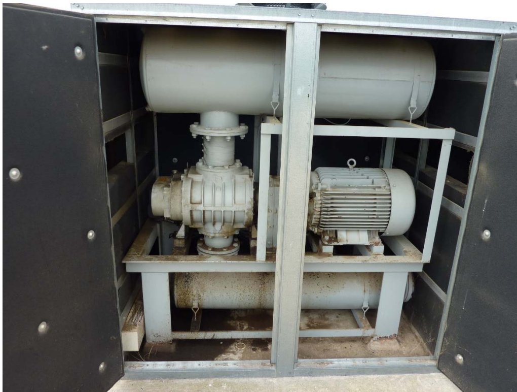
Blower Package No. 2 in sound enclosure (typ.)
