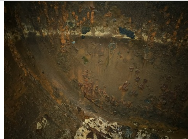
Close up of pitting on western head
