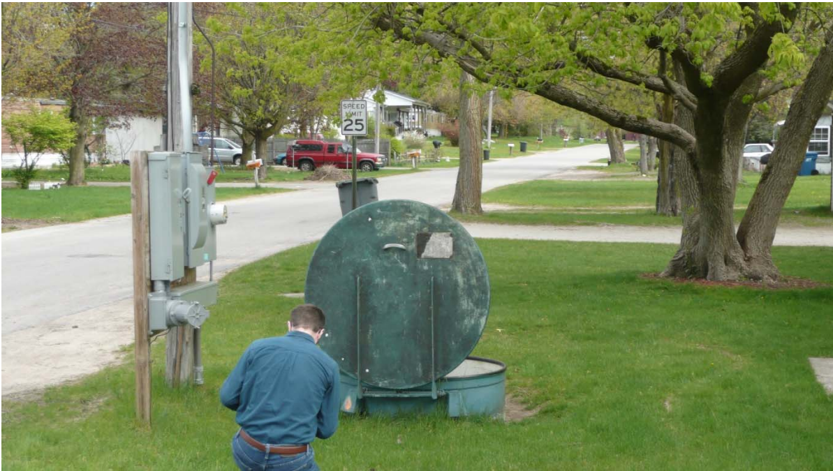
Lift Station Site
