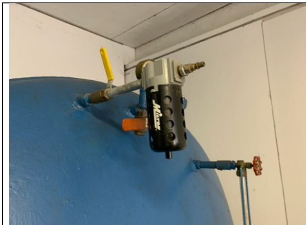
Regulator where the compressor is connected to the tank
