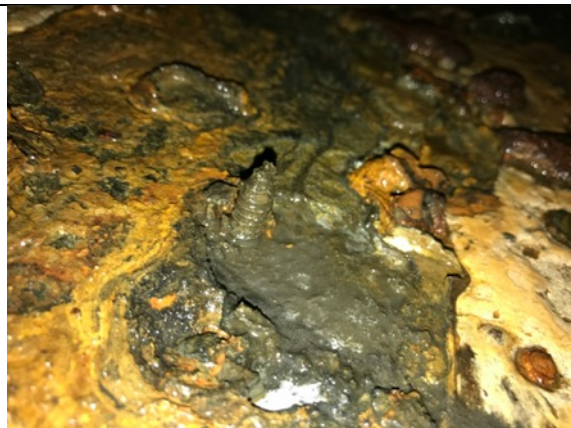
Deep pit on floor with screw repair where it pitted through
