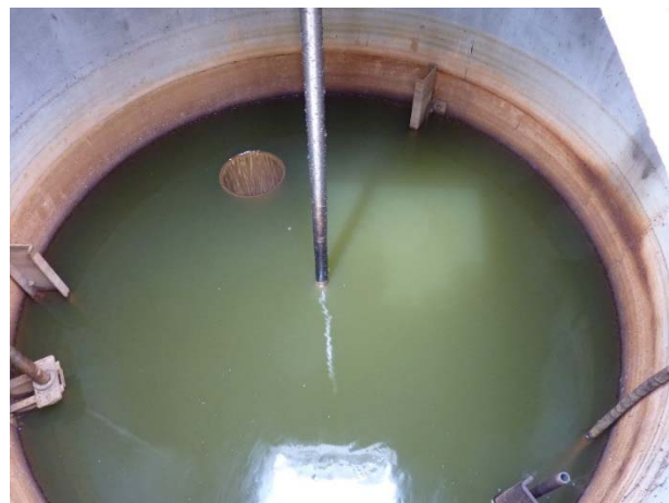
Flocculation Chamber No. 2 (M-2 shaft shown)
