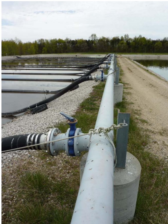
Lagoon No. 1A air header and berm (good condition) Blower No. 2 failed air relief valve
