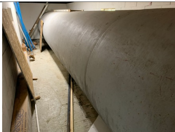
5,700-gallon hydropneumatic tank with gray topcoat in annex room
