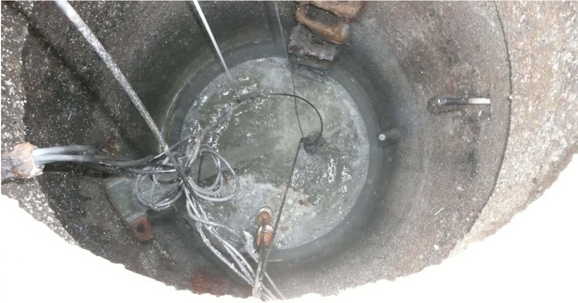
Wet Well with pitted concrete walls
