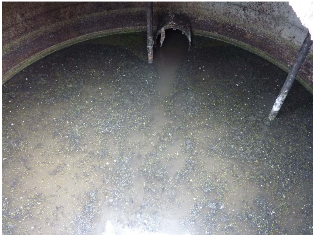
Solids carryover from Lagoon No. 1A2 in MH#1
