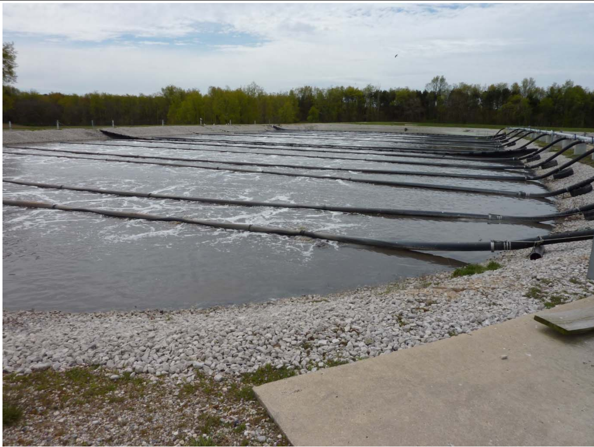
Lagoon No. 1A (facing south)
