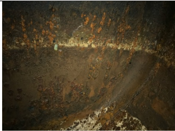
Close up of pitting on western head
