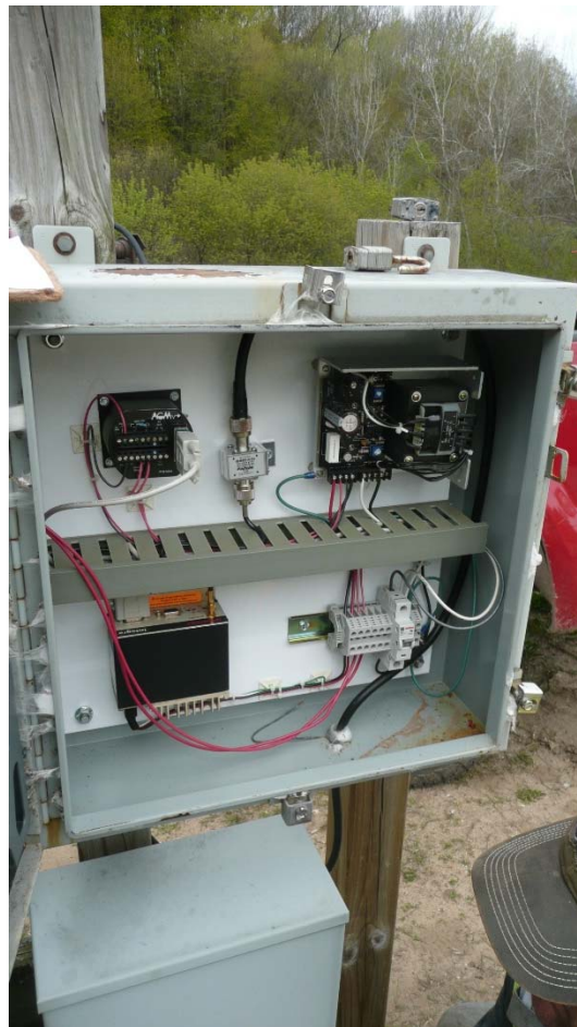
Alarm Telemetry panel
