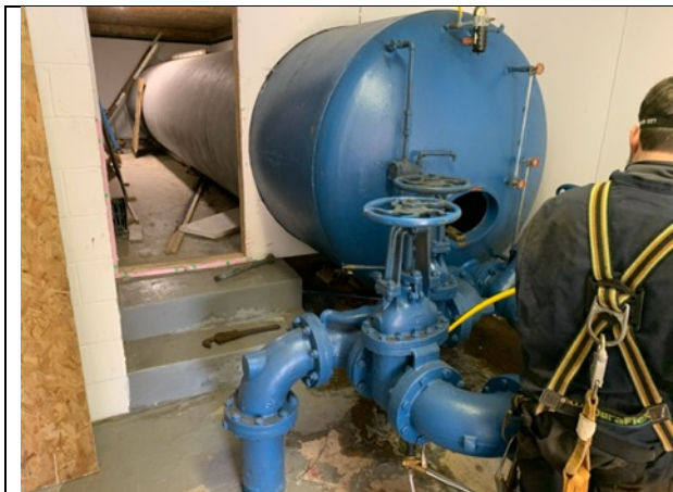
5,700-gallon hydropneumatic tank with blue topcoat in pump room
