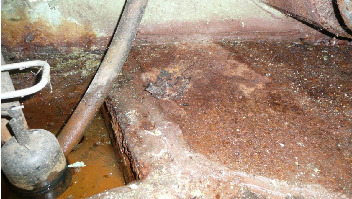
Pitting of can floor steel near sump
