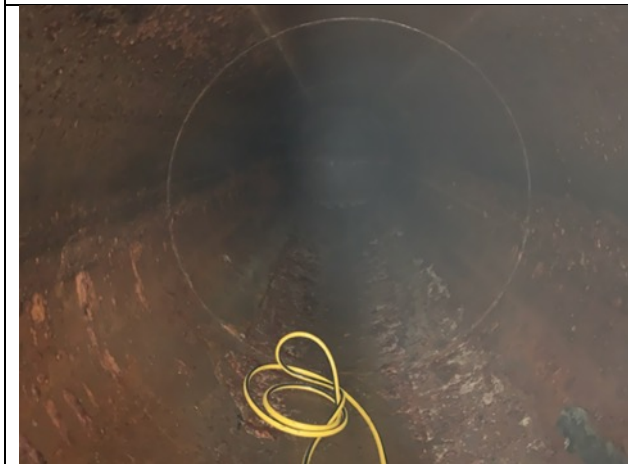
Interior tank with pitting on floor, walls and roof
