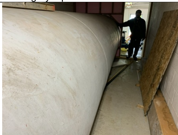
Minor chipping of the top coat
