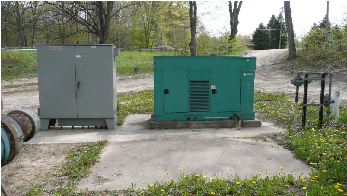
Control Panel enclosure and Standby Generator
