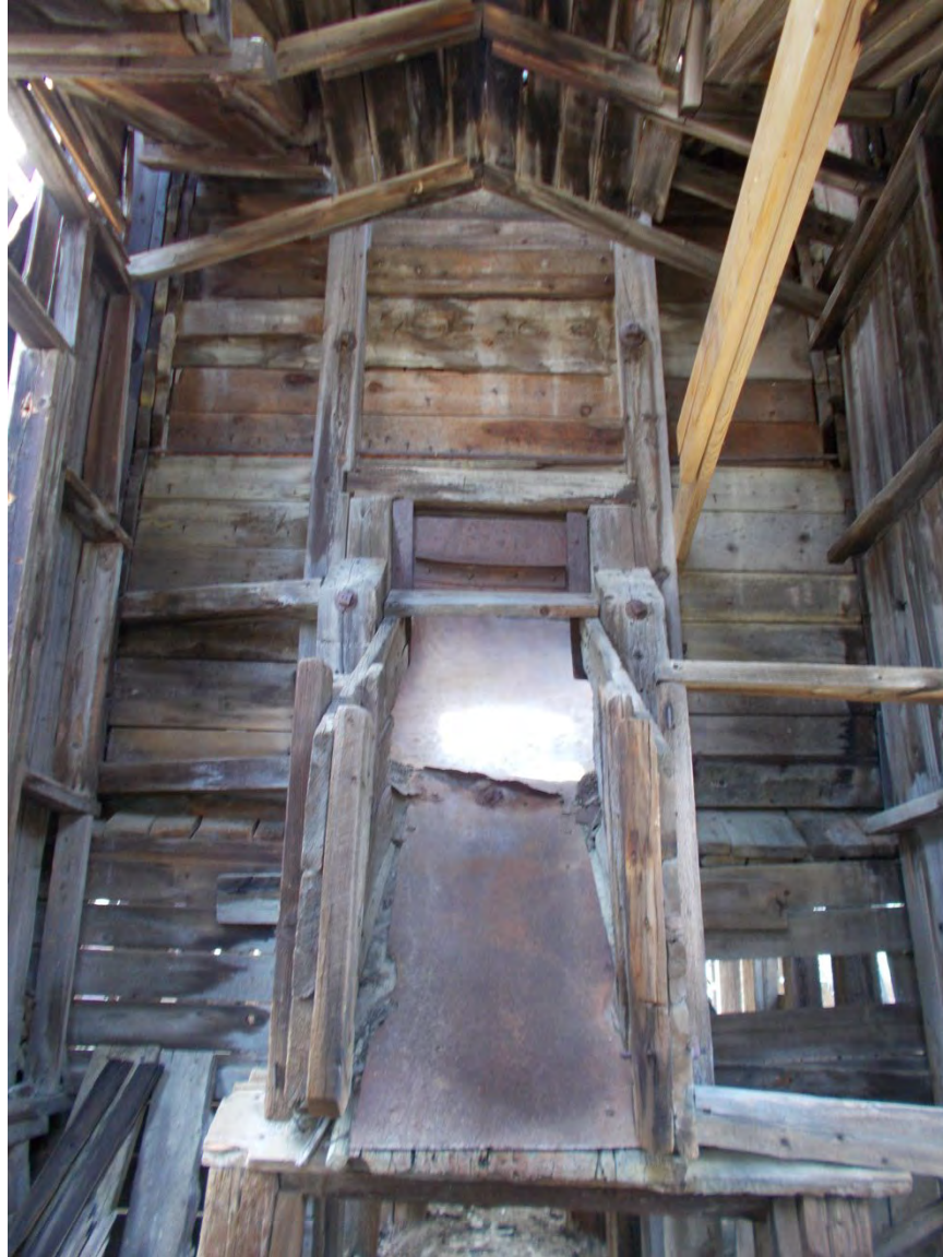
Photo 40: Detail of the central interior ore chute on the east side of the main ore bin, running into the tramway extension. View southwest.
