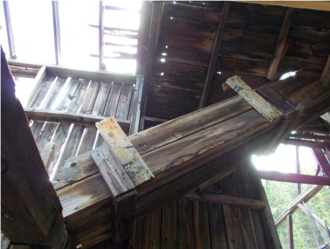
Photo 41: Detail of the interior wood ore chute located above the central ore chute, emptying into the ore bin on the south side of the tramway. View east.
