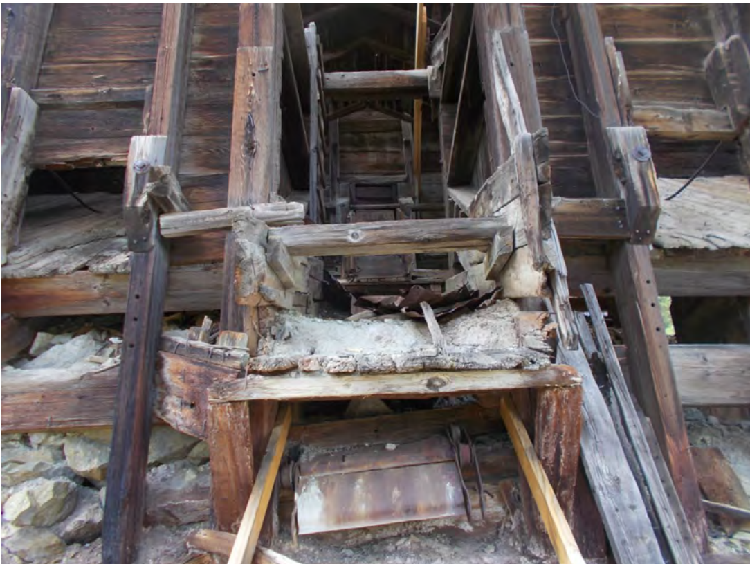
Photo 41: Detail of the interior wood ore chute located above the central ore chute, emptying into the ore bin on the south side of the tramway. View east.
