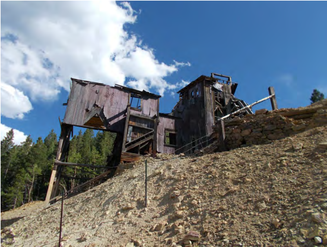
Photo 34: Oblique view of the northeast corner of the Frontenac Shaft House. Note the intact timber and stone retaining for the original 1888 Gilpin Tramway rail line photo right. View south.
