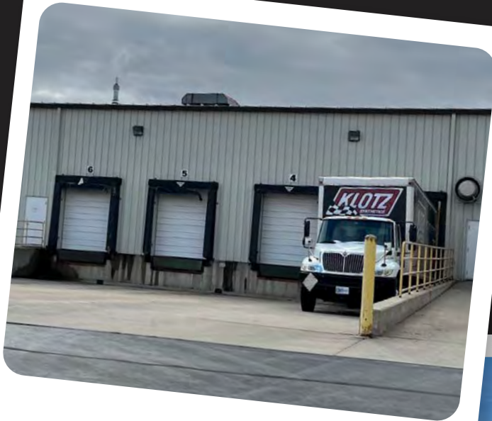
Klotz Loading Docks
