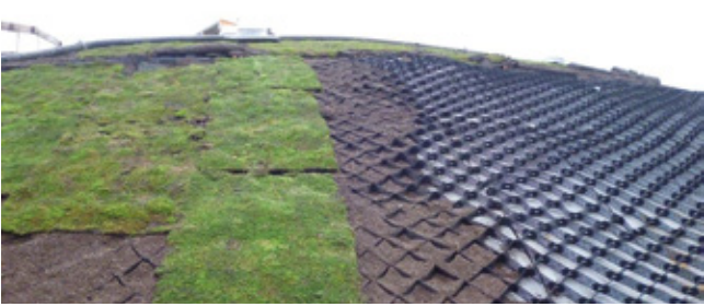
SoilWeb® Geocells and SkyGarden® Green Roof Mats
