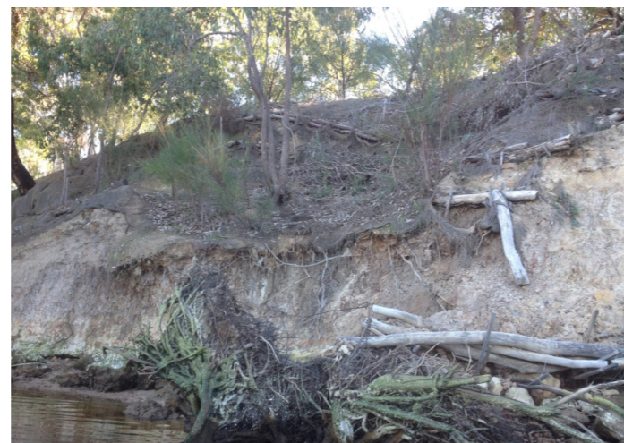
Image showing undercutting and failed superficial erosion mitigation matting
