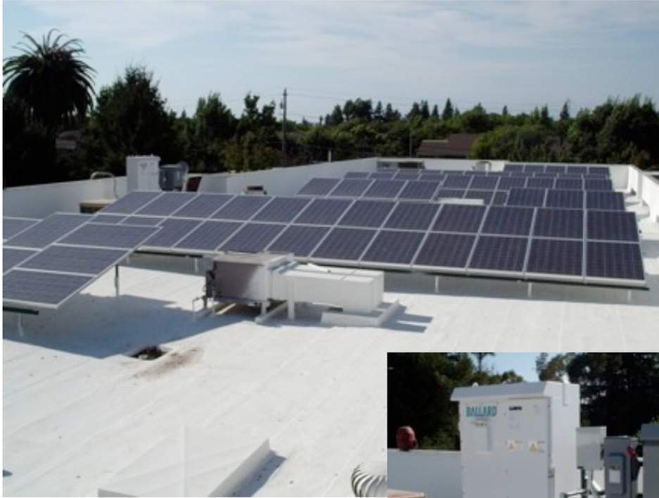
'3 Phase Inverter > Transformer & Service Panel >'
