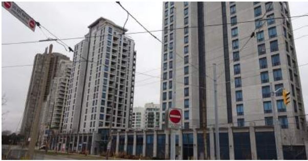
2083 – 2095 Lake Shore Boulevard West
