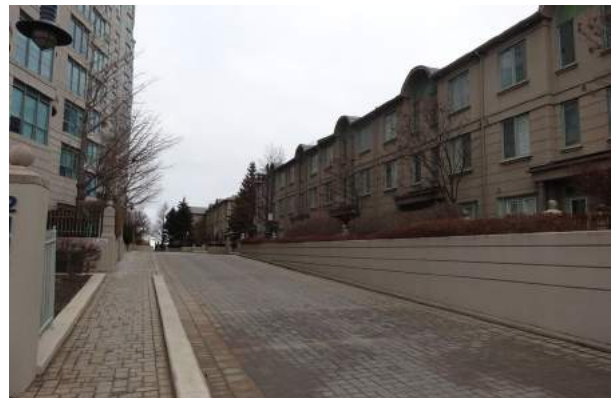
2111 Lake Shore Boulevard West
