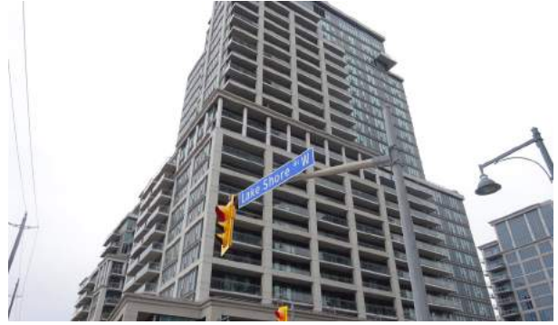
2121 Lake Shore Boulevard West
