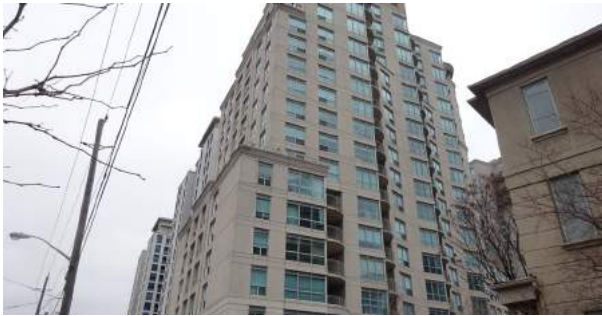
2111 Lake Shore Boulevard West
