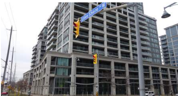
2121 Lake Shore Boulevard West
