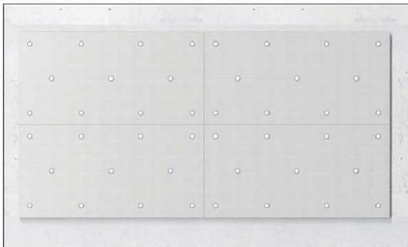
Figure 1.2. Board joints aligned. Fastener pattern
