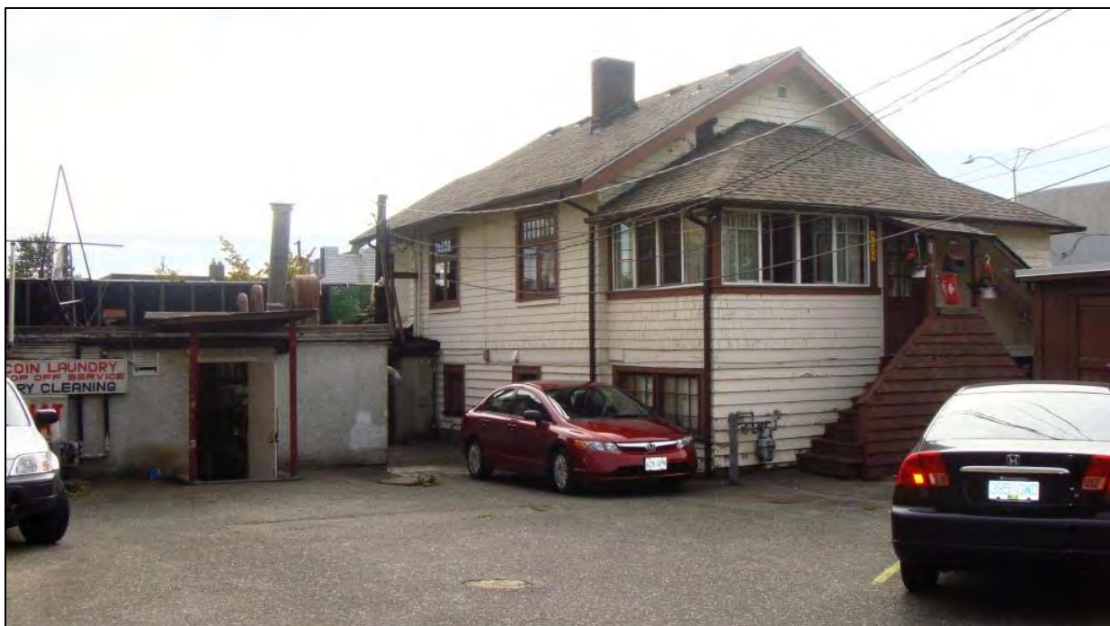
Photo 2: View of the residence, rear entrance to the laundry and parking lot. Looking SW.
