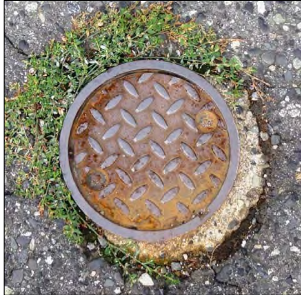
Photo 5: View of the one of three of the monitoring wells installed in 1998 and located in the central north area of the site at 4227-31 E. Hastings.
