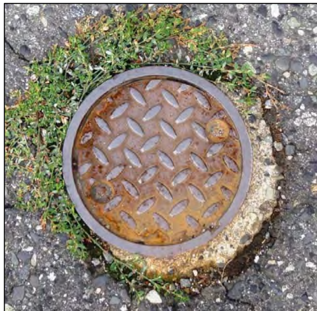
Photo 5: View of the one of three of the monitoring wells installed in 1998 and located in the central north area of the Site.
