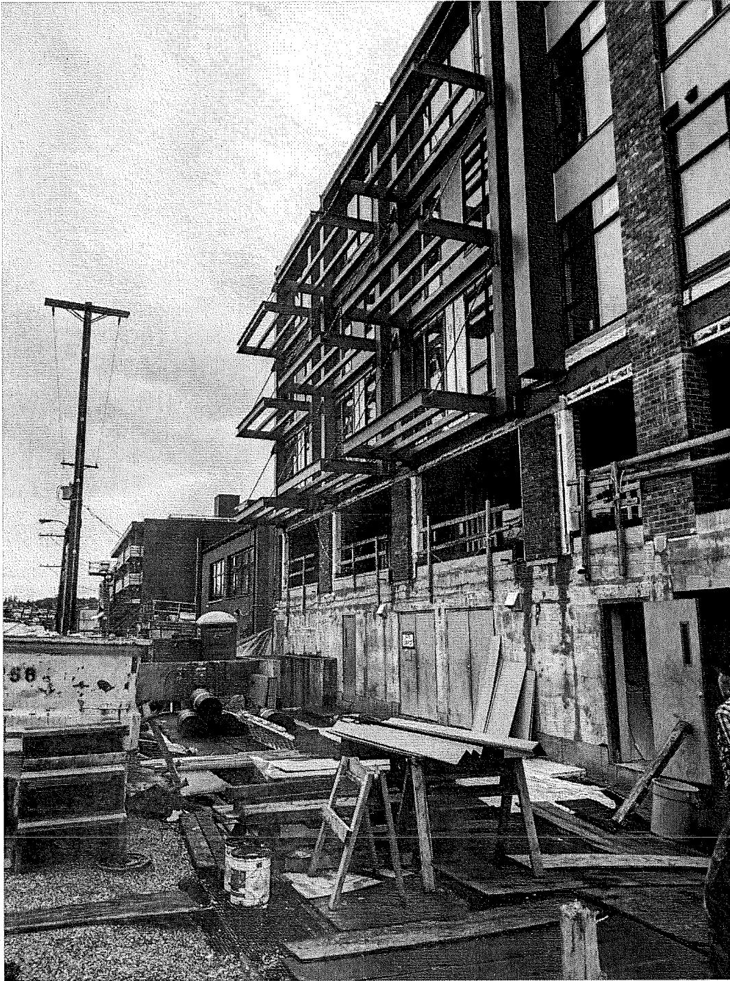
North Elevation of Building:
