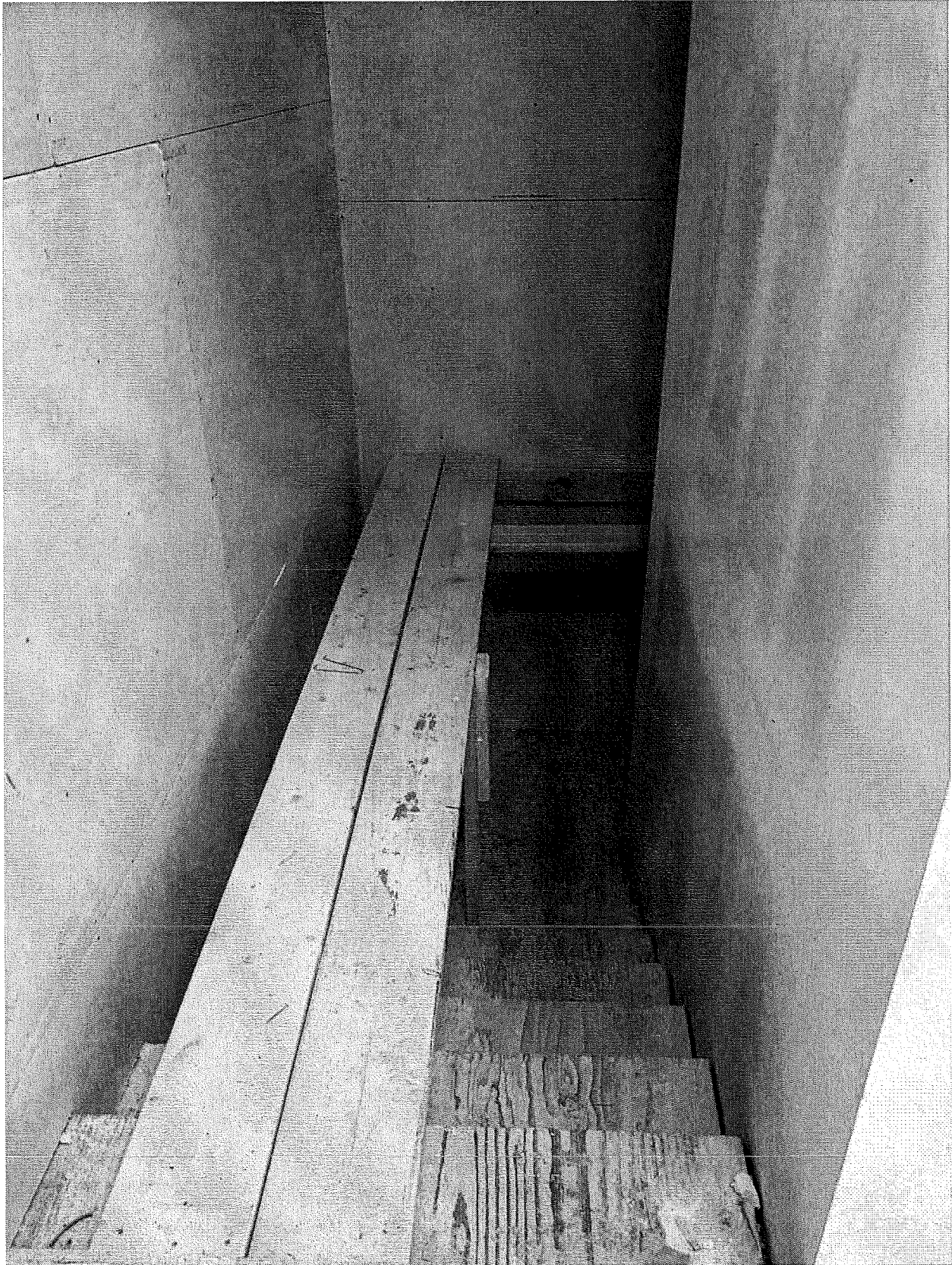
Stairs at top level:
