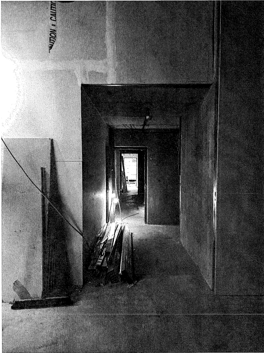
Main Lobby Looking North to access Corridor (leading to elevator):
