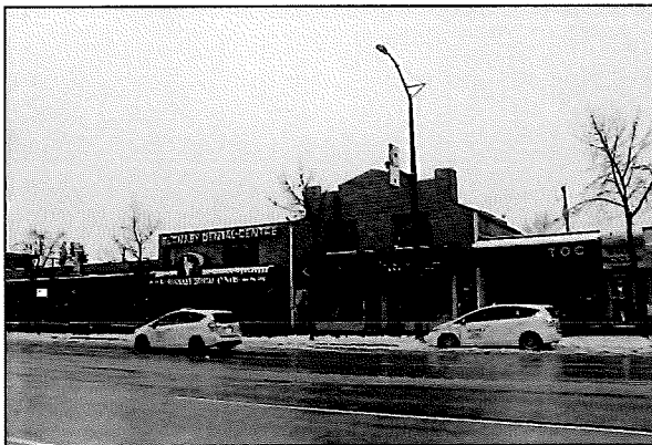
Commercial and mixed-use development opposite subject to south
