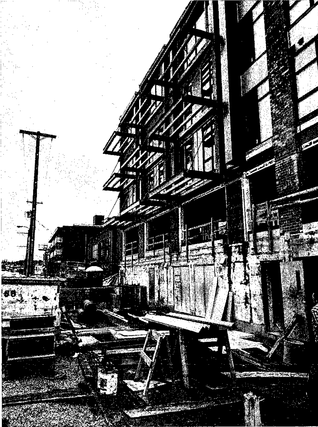
North Elevation of Building:
