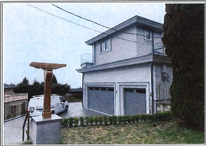
EAST WALL OF HOUSE
