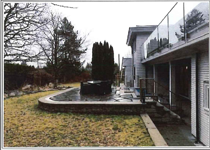
REAR YARD - NOTE BASE LEVEL OF LANDSCAPING
