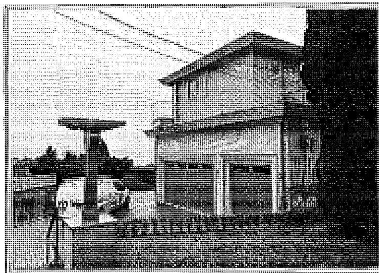
EAST WALL OF HOUSE
