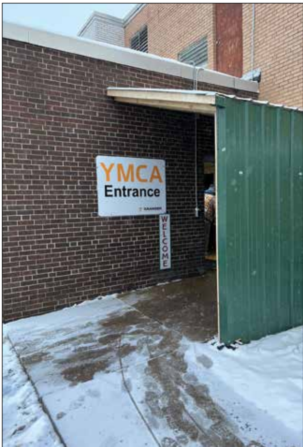
Weather barrier installed at temporary entrance to maintain a comfortable environment.
