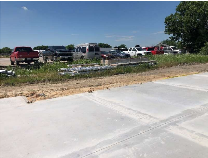
Building sheathing has also been delivered.
