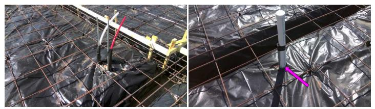
Gaps in the poly should be taped where plumbing pipes penetrate the poly.
