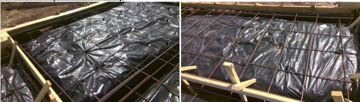
• Some of the rebar has not been adequately lifted off of the concrete pads at the back of the home. The rebar should be supported by chairs so that th rebar is fully encased in concrete.
