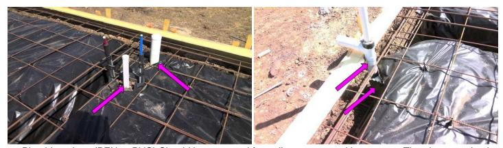
Plumbing pipes (PEX or PVC) Should be protected from direct contact with concrete. The pipes need to be
