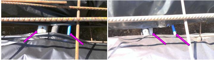
• Plumbing pipes (PEX or PVC) Should be protected from direct contact with concrete. The pipes need to be wrapped with pipe insulation or at minimum 8 mil poly so that they do not come into direct contact concrete. This also helps to protect plumbing pipes from seasonal foundation movement.
