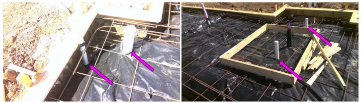
Plumbing pipes (PEX or PVC) Should be protected from direct contact with concrete. The pipes need to be
