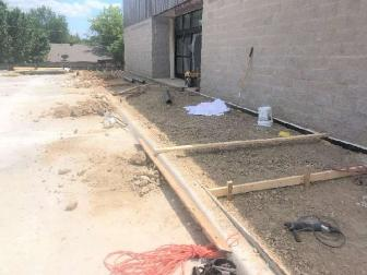
• The sidewalk near the front and side of the building was formed up and getting ready to be poured.
