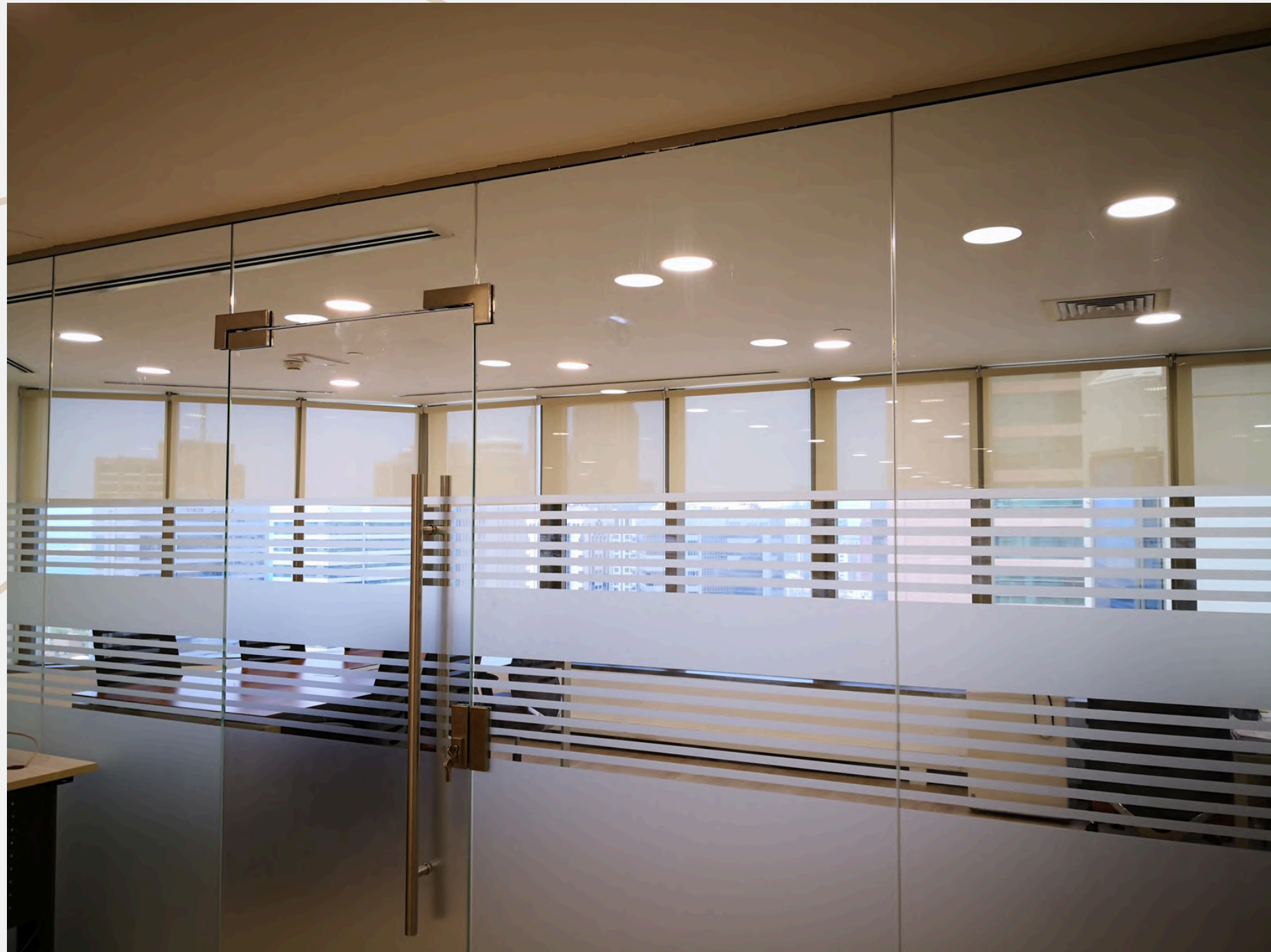
Glass partition installation
