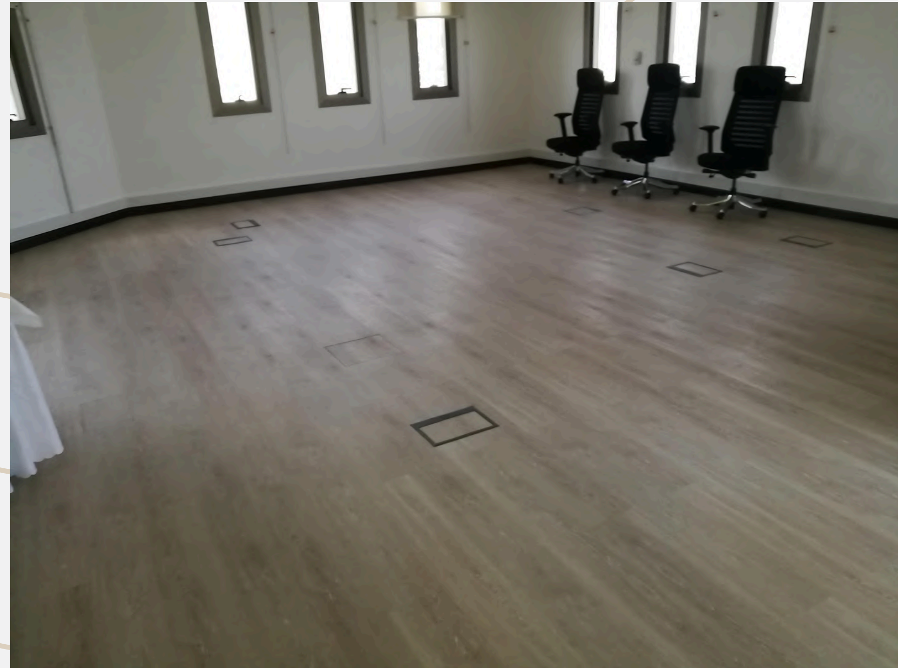
Parquet Flooring Installation
