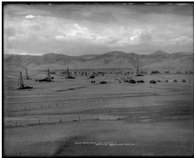
Five oil derricks can be seen in this oil field near Boulder between 1901-1920. A horse grazes in front of some small cabins at the right. The wood frame buildings were residences for workers. Oil storage tanks and a production facility can also be seen. Courtesy of Denver Public Library
