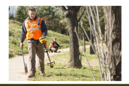
All new underground facilities, including laterals up to the structure or building being served, installed after August 8, 2018 must be electronically locatable when installed.
