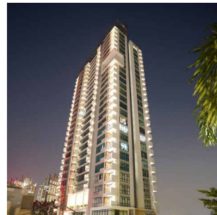
VERANDA RESIDENCE PURI, JAKARTA
