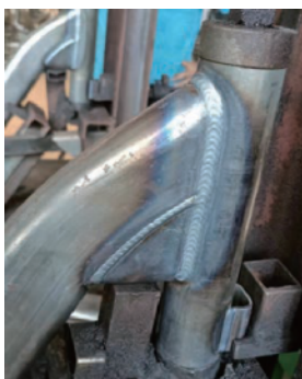
▶ Quick Spot Welding
