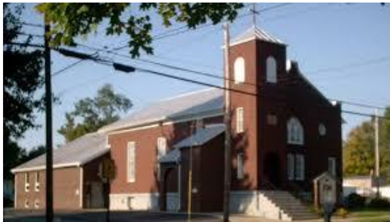
The picture above shows the side of the church and the addition that was put on the back of the church
