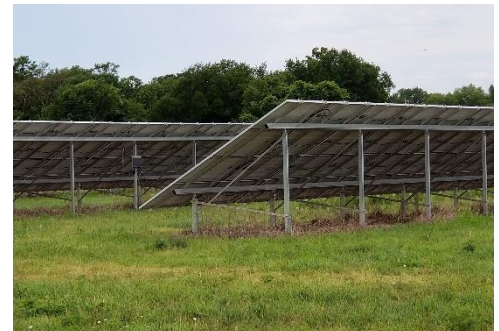
Example of a Solar Conversion System, Ground-mounted
