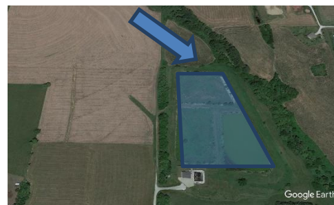
City of Bennet wastewater lagoon
