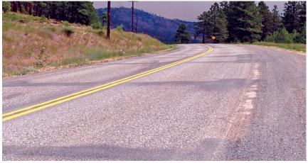
An example of spray patching used to treat transverse cracks. This is an example of poor spray patching, as the ride was not improved because the patching created bumps.
