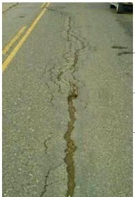
Possible Types\* Longitudinal Wheel Path Cracking (LWP), Longitudinal Joint Cracking (LJC), Meandering Longitudinal Cracking (MLC), Most Likely Cause Frost heave, poor joint construction (LJC), heavy traffic (LWP), and construction problems (MLC) Possible Repairs Crack Treatment or Spray Patching (if cracks are > 35 mm in width) Notes: The difference between these cracks is location. All can be caused by frost heave, plus each has
