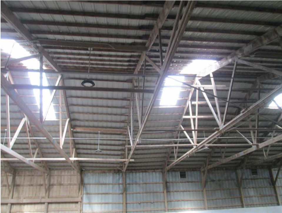
Photo 1 Sloping Roof at West Barn
