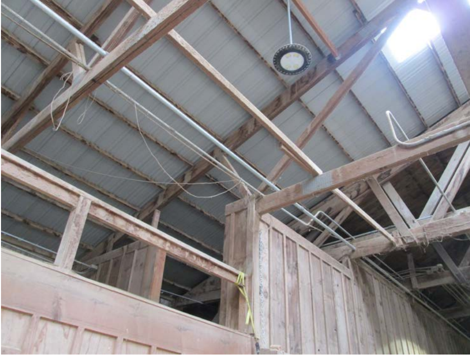
Photo 3 Cut Truss Bottom Chord Adjacent to Arena Judging Platform
