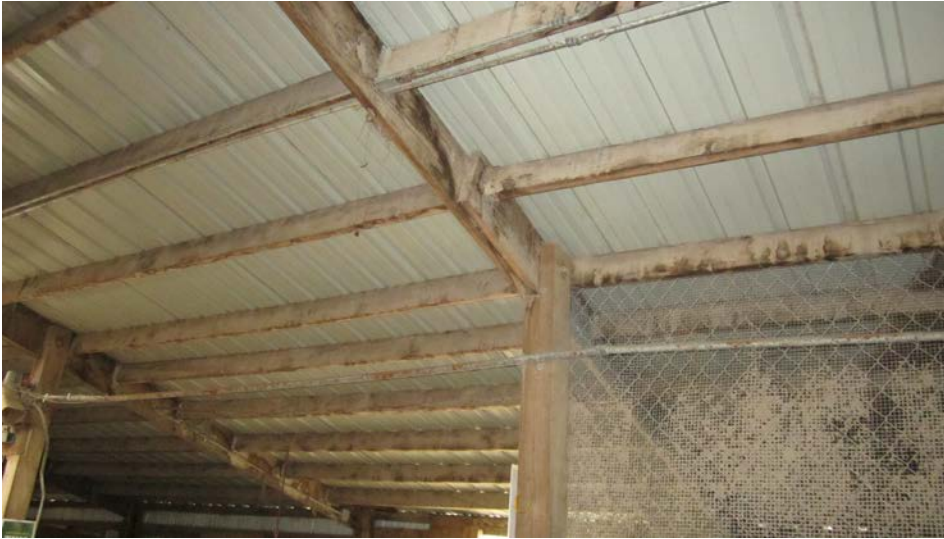
Photo 1 2x10 Roof Beam at Stable Area
