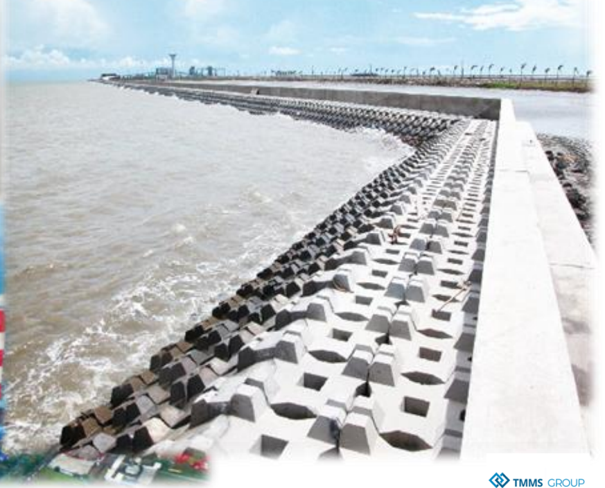
Revetment for Guangdong – Hainan Railway Project
