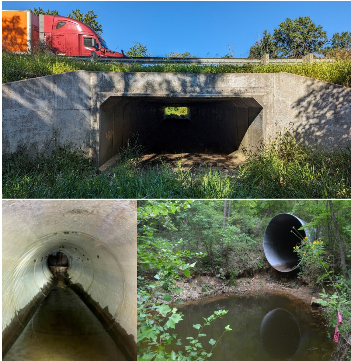
FIGURE 8. Representative culvert structures of various types, including a box culvert in Indiana (top; photo by USFWS); a round, concrete pipe culvert design in Georgia (bottom left; photo provided by Georgia Department of Natural Resources); and a corrugated metal pipe culvert design in Missouri (bottom right; photo provided by L. Droppelman).
