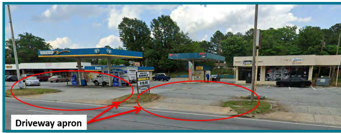
Figure 5-7: Driveway Aprons along Riverdale Road
