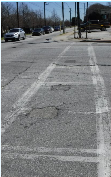
Surface potholes, blurry crossing lines at the street crossing
