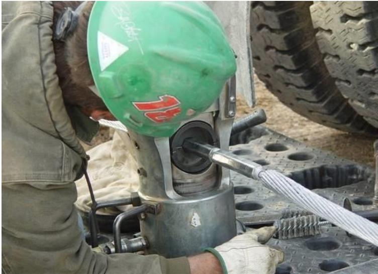
Secure the forging assembly to the rigging to not allow the conductor to be dropped. This can put stress on the 3M ACCR core wires.
