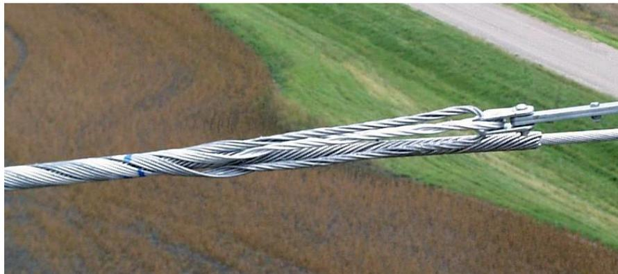
After the final sag tension of the conductor is established, a measurement is made on the conductor to determine where the dead-end assembly will connect to the insulator string. There are two layers that make up the construction of the preformed dead-end assembly. Each layer has match markings on them. These match markings will determine where the first layer of reinforcement rods will be placed onto the
