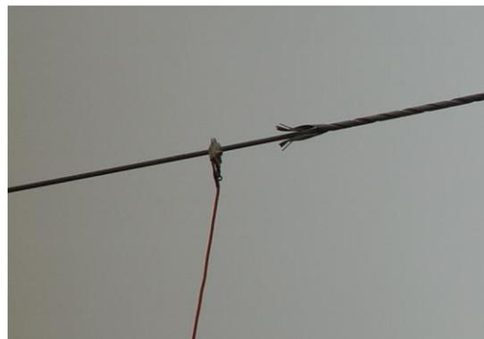
**Conductor Grounding Clamp**
