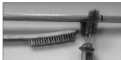
FIGURE 2: Clean a distance of at least \frac{3}{4} the distance of the aluminum dead end body.
