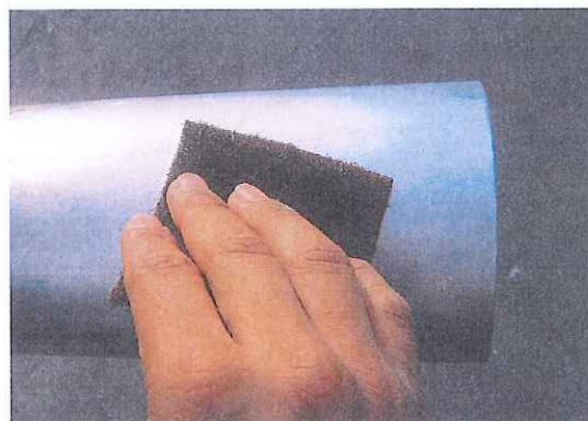
Figure 2: Cleaning the bus with a rough cloth.
