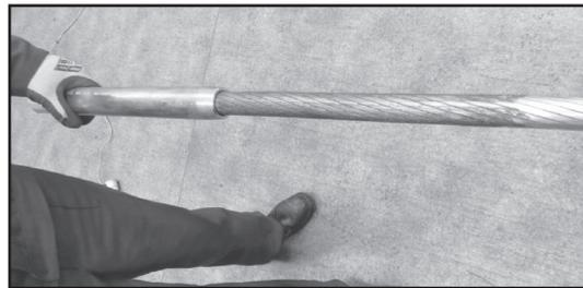
**Step #8** Apply the oxide inhibitor to the outer surface of the inner aluminum sleeve, excluding the tapered section.
