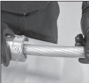
**Step #2** Apply the supplied oxide inhibitor along the length of the wire brushed aluminum strands.
