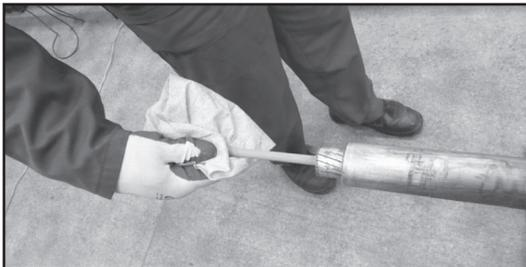
**Step #5** Clean/wire-brush the entire aluminum area to be covered by the compression hardware per your standard company practices. Check that no residue or surface particles remain.
