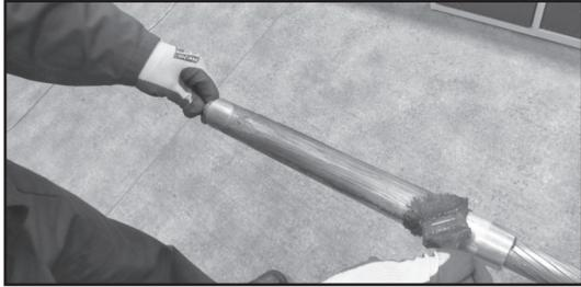
**Step #9** Slide the outer aluminum dead-end sleeve over the ACCC conductor toward the filler tube.
