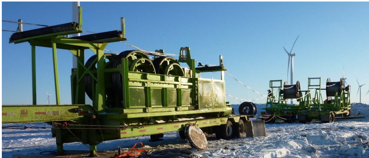
Figure 6. Payoff and bullwheel setup.
