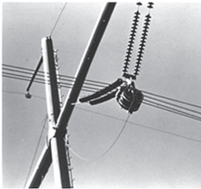
a) Application of traveler ground
