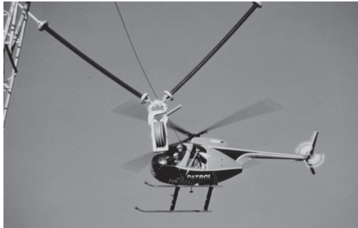
Figure 18—Helicopter installing pilot line
