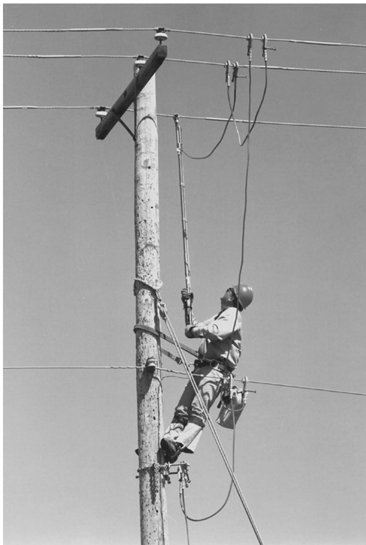
Figure 13.1 A grounding cluster installed on four-wire, three-phase line. The line conductor mounted on side of pole is the grounded neutral conductor. The grounding conductors create a low-impedance short circuit around the line-man's work area. (Courtesy of A. B. Chance Co.)
