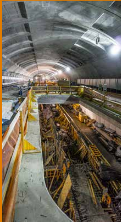
SECOND AVENUE SUBWAY
