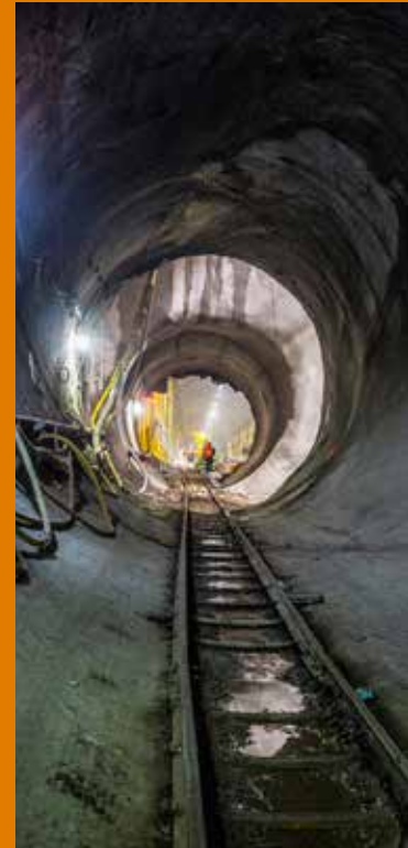
EAST SIDE ACCESS
