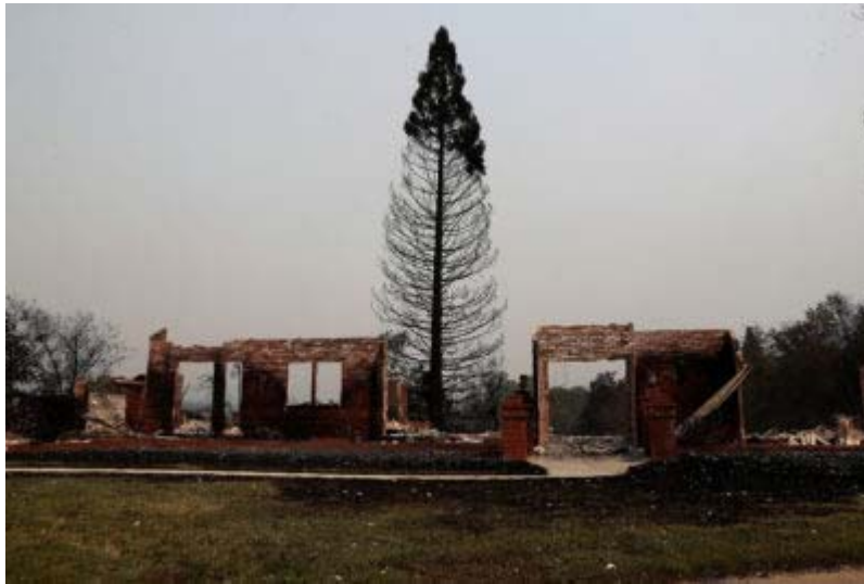
A home in Redding destroyed by the Carr Fire. (Justin Sullivan/Getty Images)
