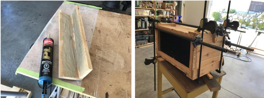
Corners glued together with PL300 and clamped overnight (24 hours).
