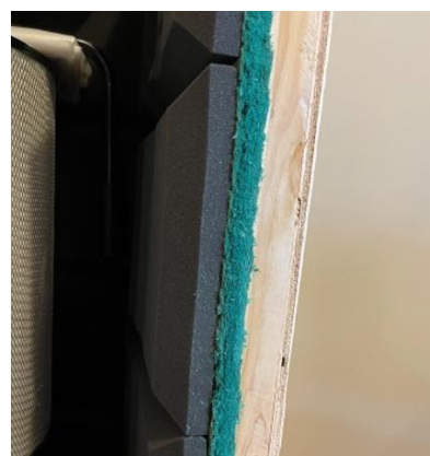
Sound proofing (combination of composite board and acoustic foam tiles).
