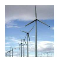
Wind is another natural resource that will always be available. Windmills have arms that turn in the wind. When the arms turn, the windmill changes wind energy into electrical energy. Windmills are built in special places that have lots of wind. When many windmills are built in the same place, we call that place a wind farm.
