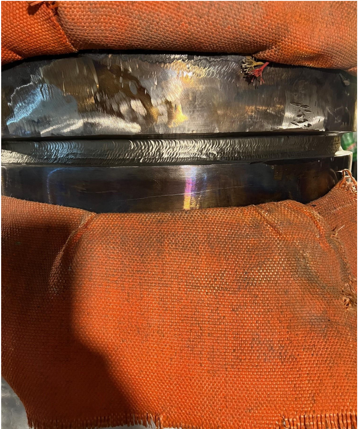
Pipe joint with a tig root/hot and some tig fill passes.
