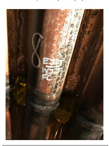
The welders stencil number for this tube was **EJ-T** and **WJ-T**. Often welders will write R/F/C or a combination of R, F or C in the area around their stencil to communicate that they only put in a root, fill or cap in the event of night shift finishing a weld that day shift started or vice versa.
