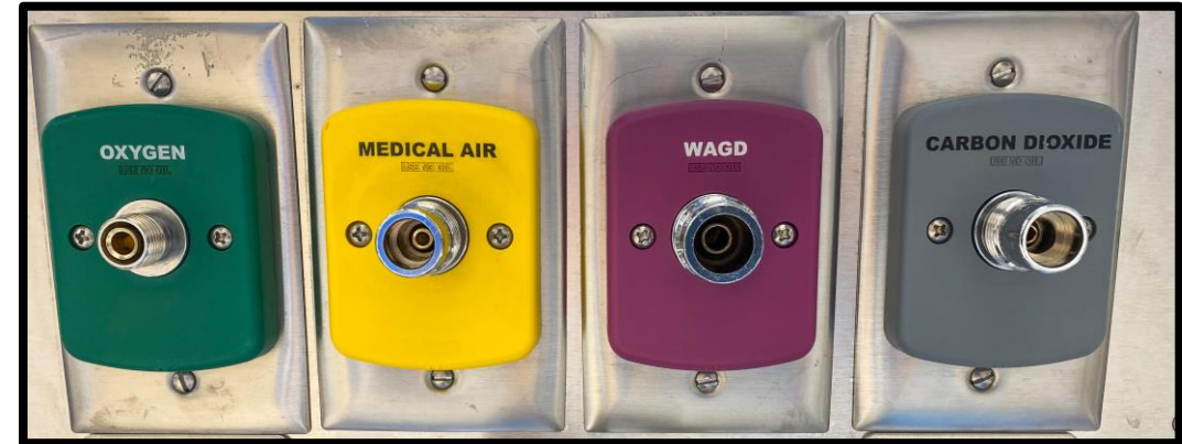
Diameter Index Safety System
