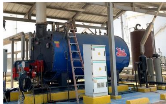
Oilon GKP 240 M WD100 Gas natural / Diesel
