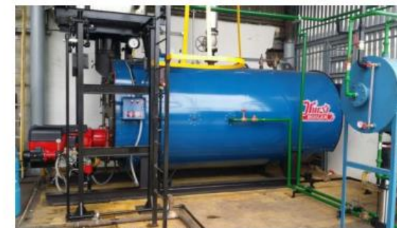
Oilon GKP 280 M WD100 Gas natural / Diesel
