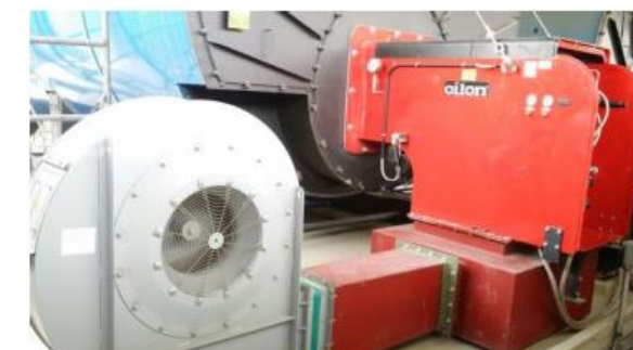
Oilon GKP 1200 M WD100 Gas natural / Diesel
