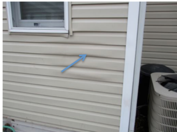
Examples of siding and trim damage at the rear of the house
