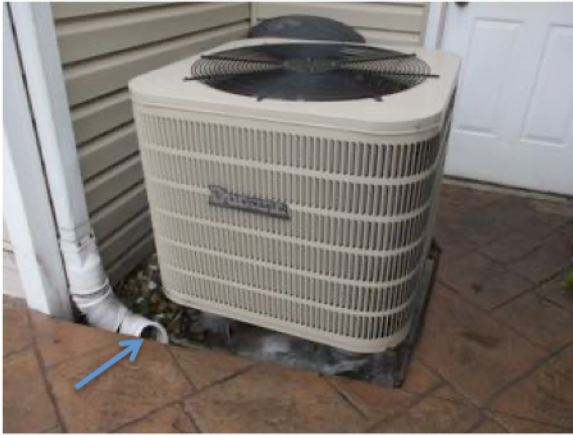
Revise downspouts to discharge further away from the house
