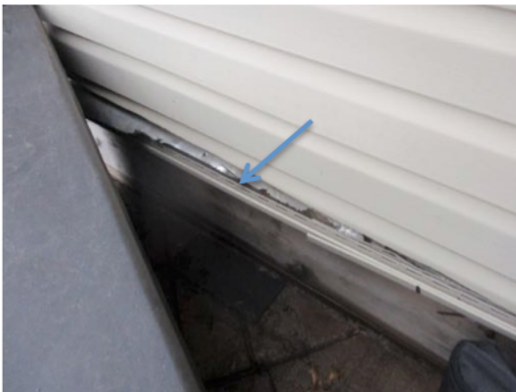
Examples of siding and trim damage at the rear of the house
