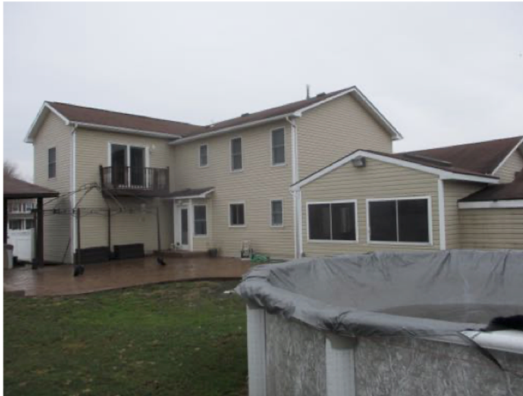
Rear view of the house
