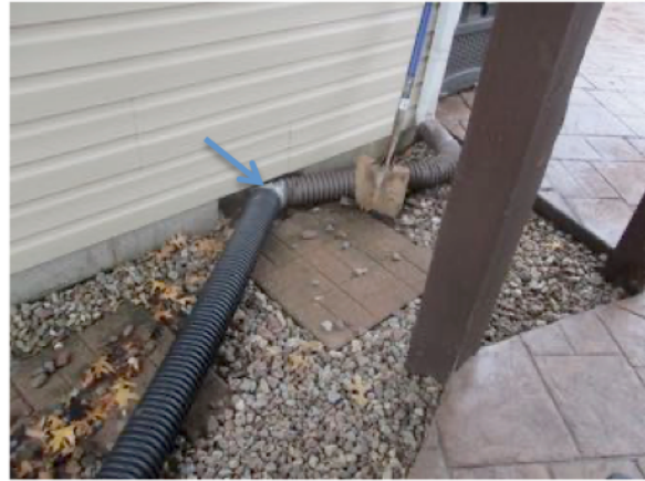
Revise downspouts to discharge further away from the house
