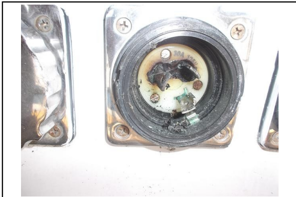
Shore Power Inlet 1
