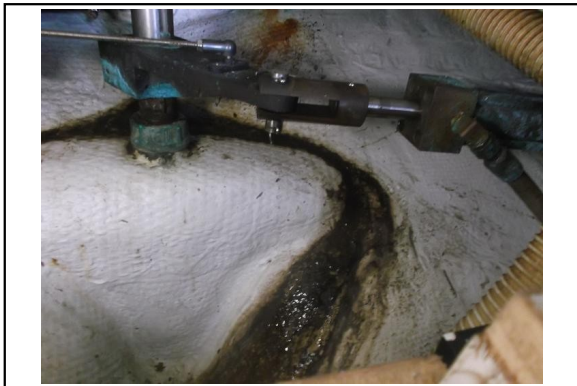
Leaking Rudder Post
