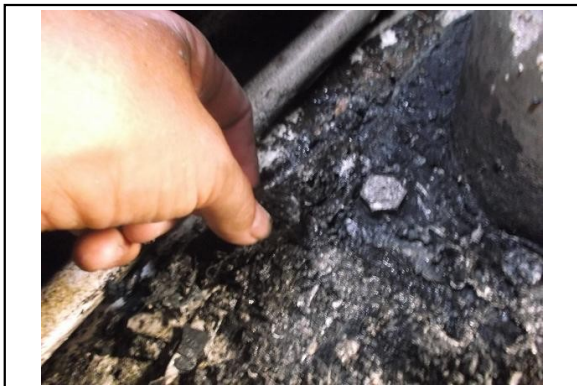
Main Mast Step
