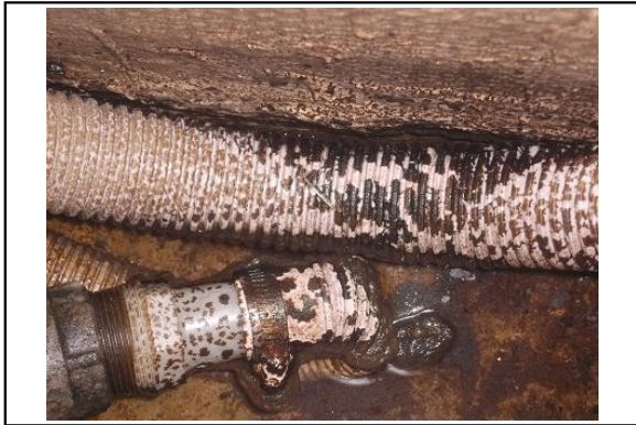
Aft Bilge Pump Discharge Hose
