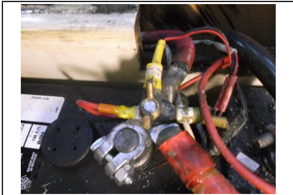
No Overcurrent Protection
